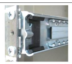
5) Install FLANGE MOUNT STATIONARY SECTION to cabinet using 10-32" screws and hex nuts. Apply to front and rear sides.
